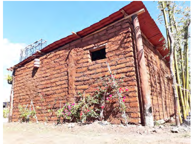
House built with bricks made of Sargassum (Sargablocks) by Omar Vazquez Sanchez in Mexico, 2019 © BlueGreen
